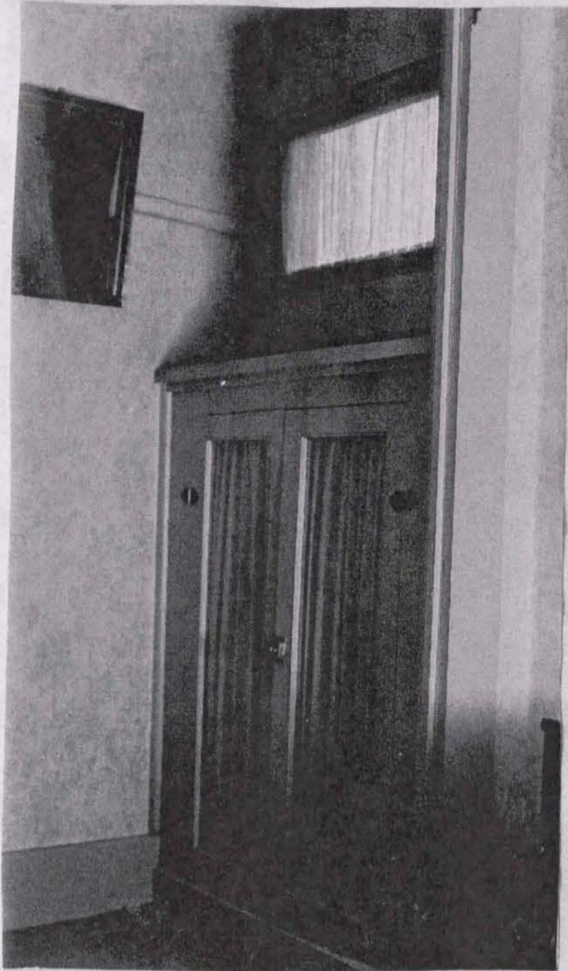
ONE OF THE SMALL WINDOWS FROM OVER THE FIRE PLACE AND THE BOOK CASE FROM THE DINING ROOM WERE PLACED IN THE BEDROOM CLOSET.
