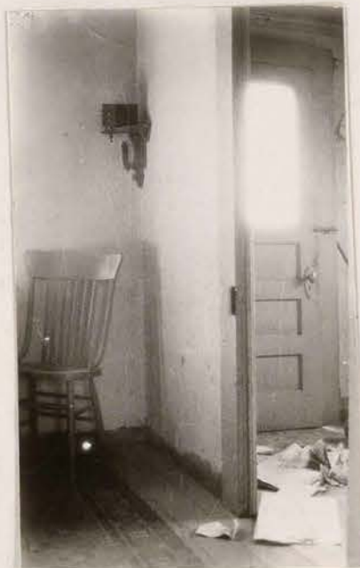
No. 7 Showing partition between kitchen and dining room
