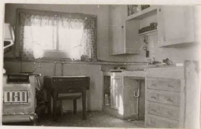
No. 11 View of same window, with new cupboards and shelves
