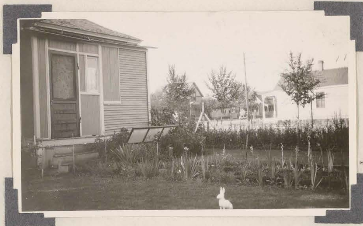
Figure 3. View of side of grounds.
