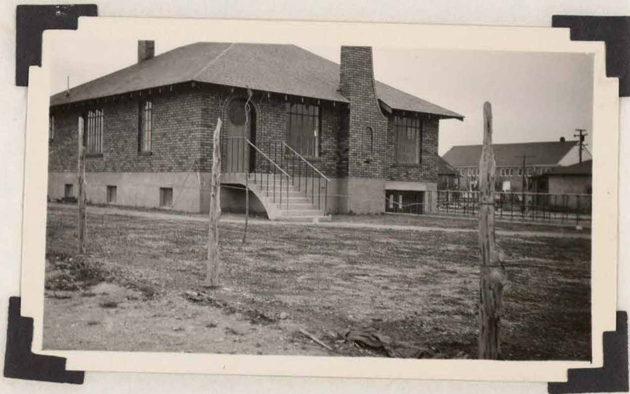
Figure 26. View showing front of grounds.
