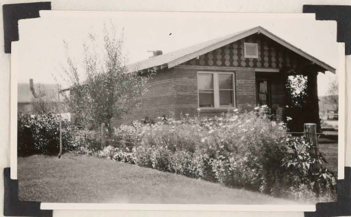
Figure 19. View from front of yard.
