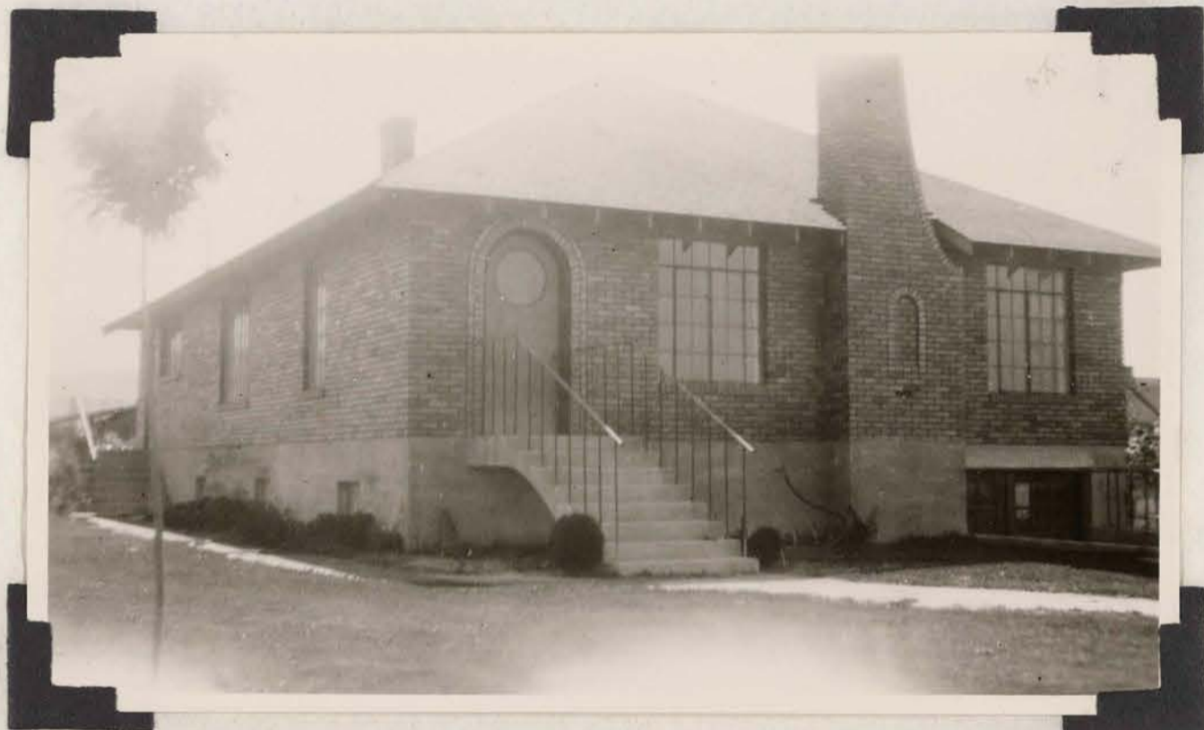
Figure 28 View showing front of grounds.
