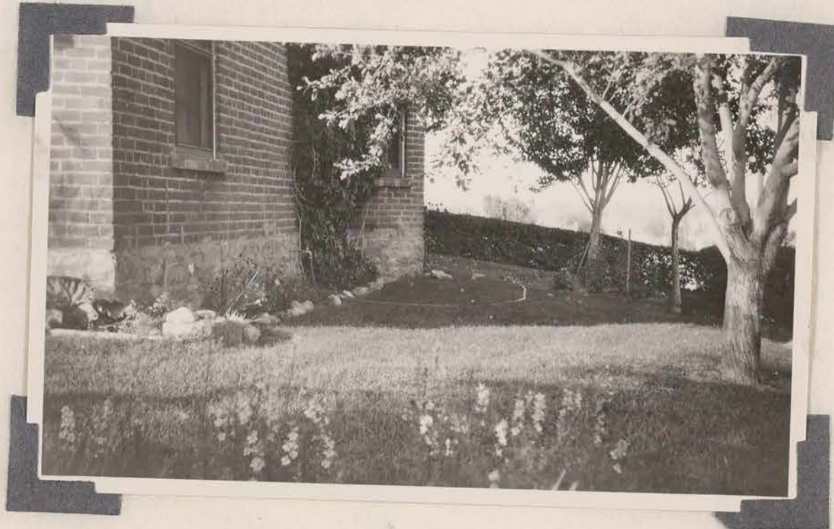
Figure 6. View of side of grounds.
