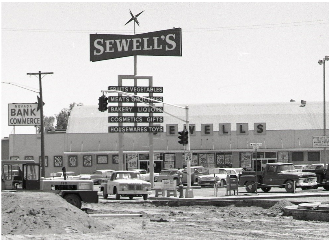
Before Statewide Lighting, the building housed Sewell's Supermarket. Nevada Department of Transportation photo.
