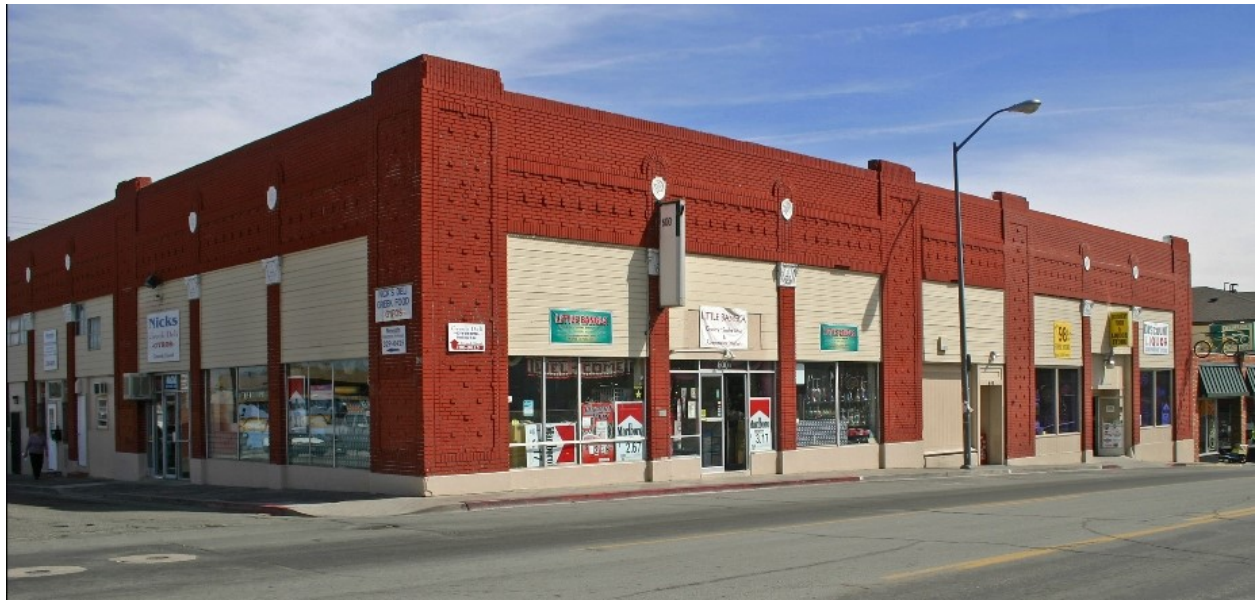
The historic Osen Motor Sales building at 600 South Virginia Street. Alicia Barber photo.
