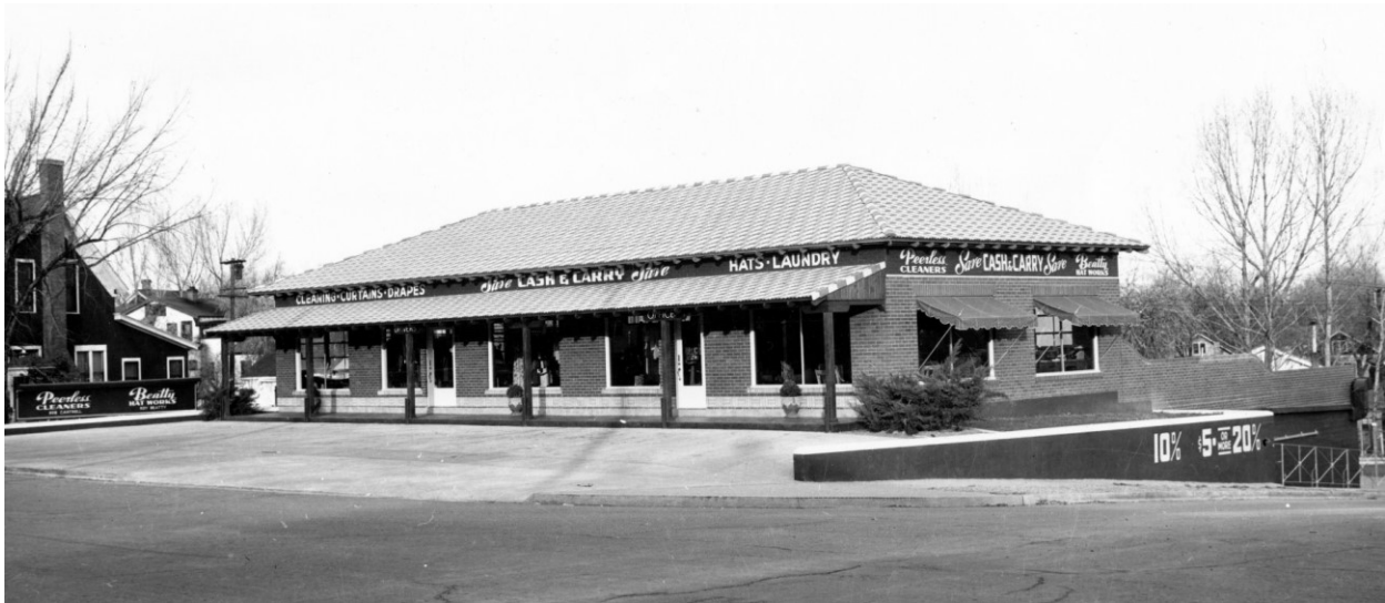
Peerless Cleaners and Beatty Hat Works opened at Forest & St. Lawrence in 1947. Mark Bonnenfant photo.
