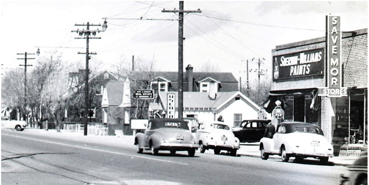
Sherwin-Williams, once located at 1460 South Virginia Street. Nevada Department of Transportation photo.
