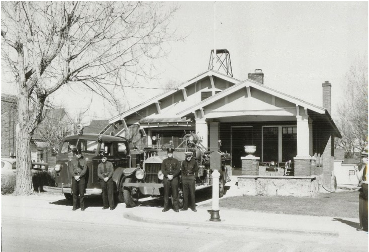
The Southside Fire Station, which once stood at 532 South Virginia Street. Photo courtesy of Joe Granata.
