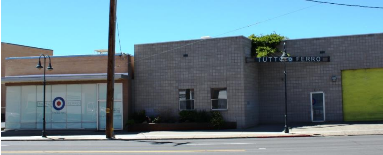
Paolo Cividino's Tutto Ferro building as it appeared in 2013. Photo courtesy of Alicia Barber.
