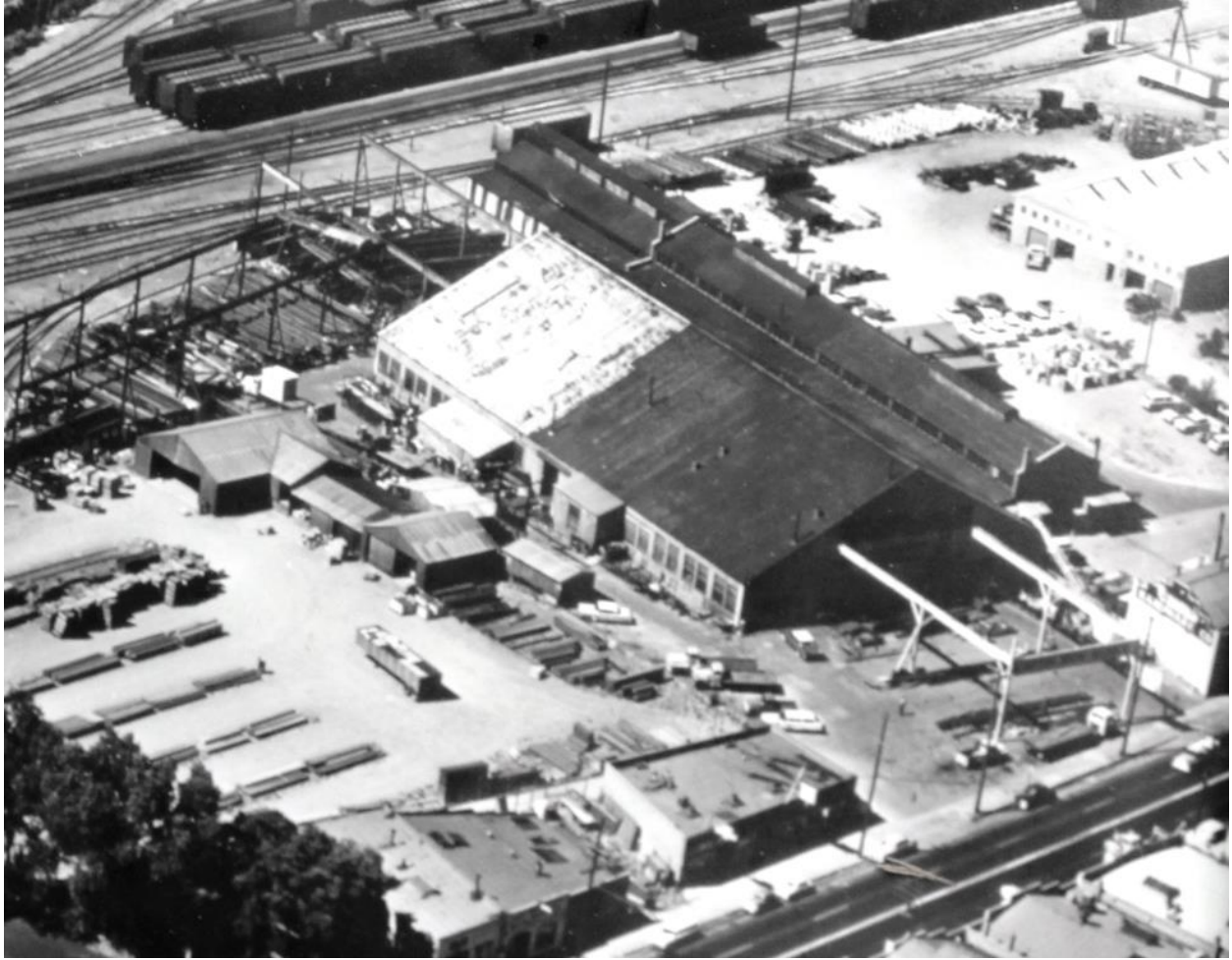
With 4th Street at the bottom of the photo, an aerial view of the Martin Iron Works site shows the original A-frame construction of the main shop building before a fire in 1962 that required the entire section to be rebuilt. Image courtesy of the Piero Bullentini family.
