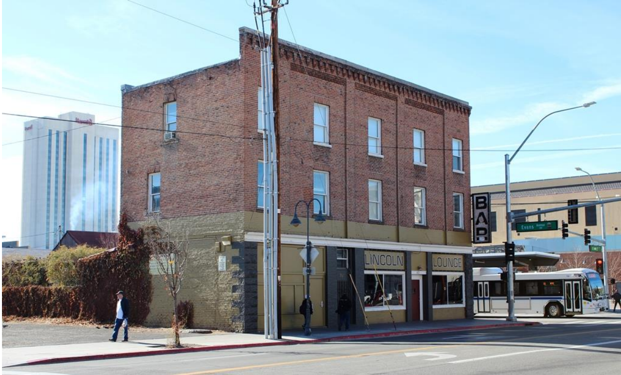
The Marion Hotel, currently home to the Lincoln Lounge, was constructed at 306 East 4 th Street in 1907. Photo courtesy of Alicia Barber.
