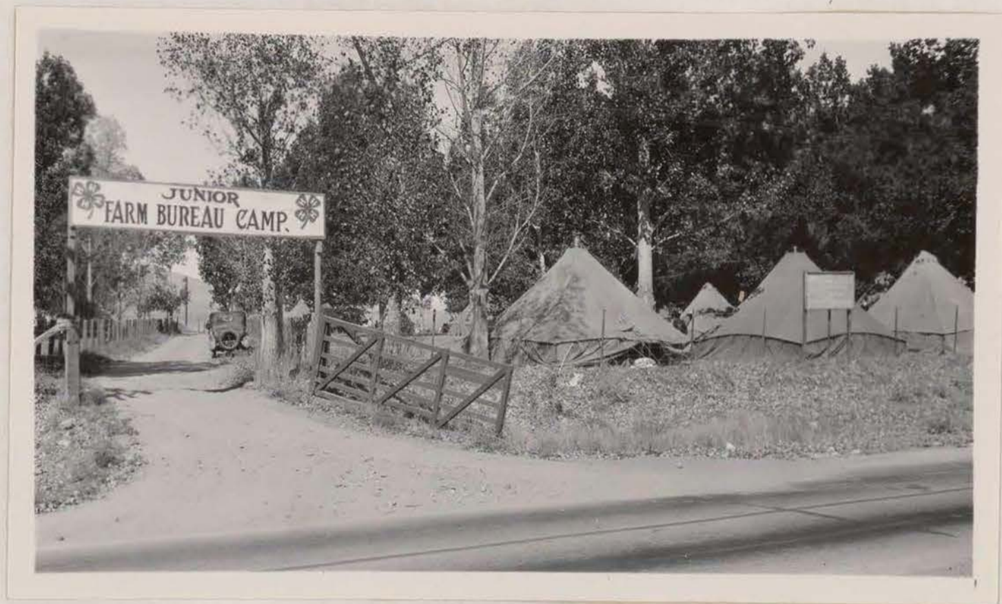
I. The Camp Site ready and waiting on Monday, August 17
