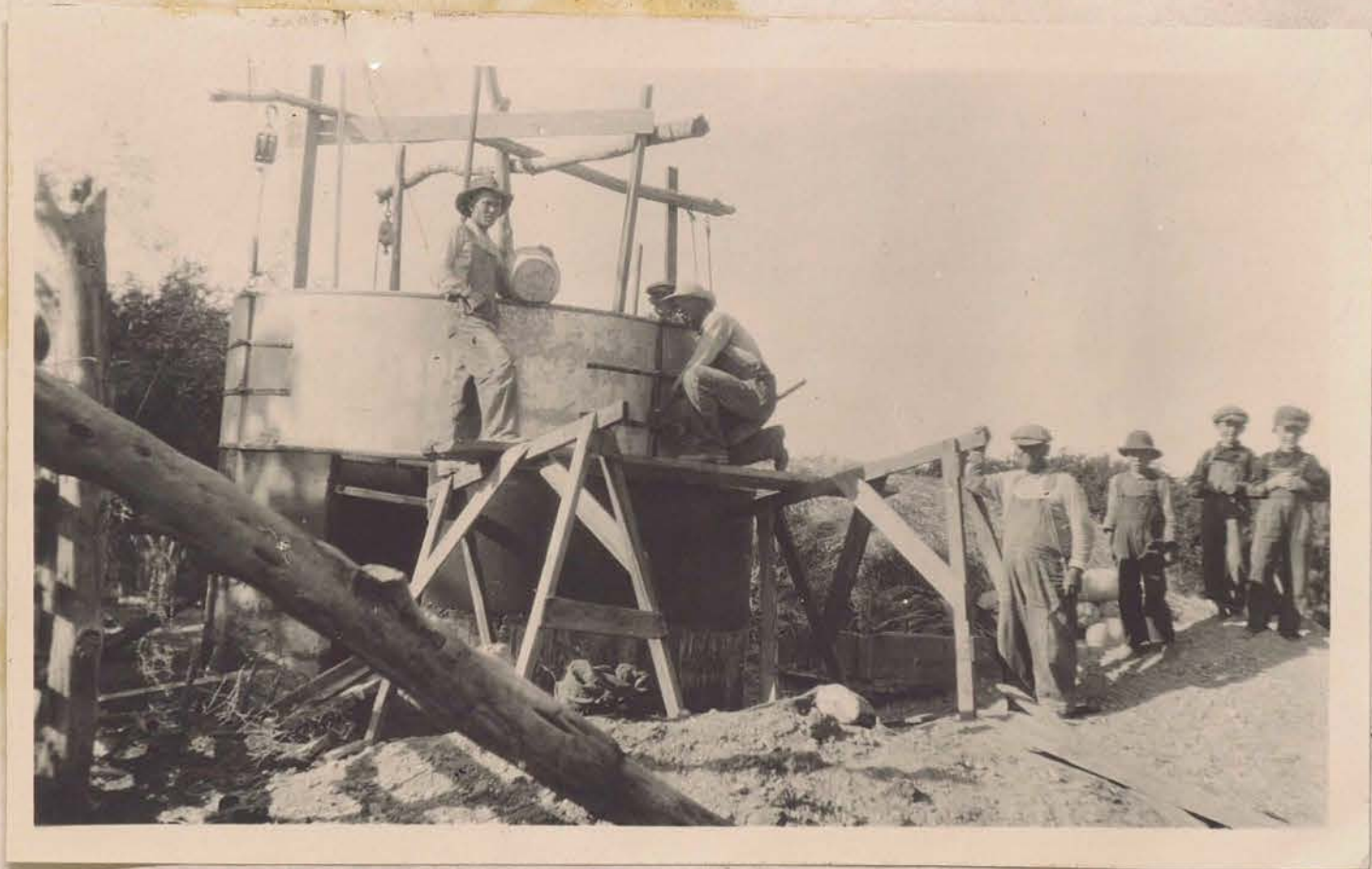
Waite Silo under course of Construction.
