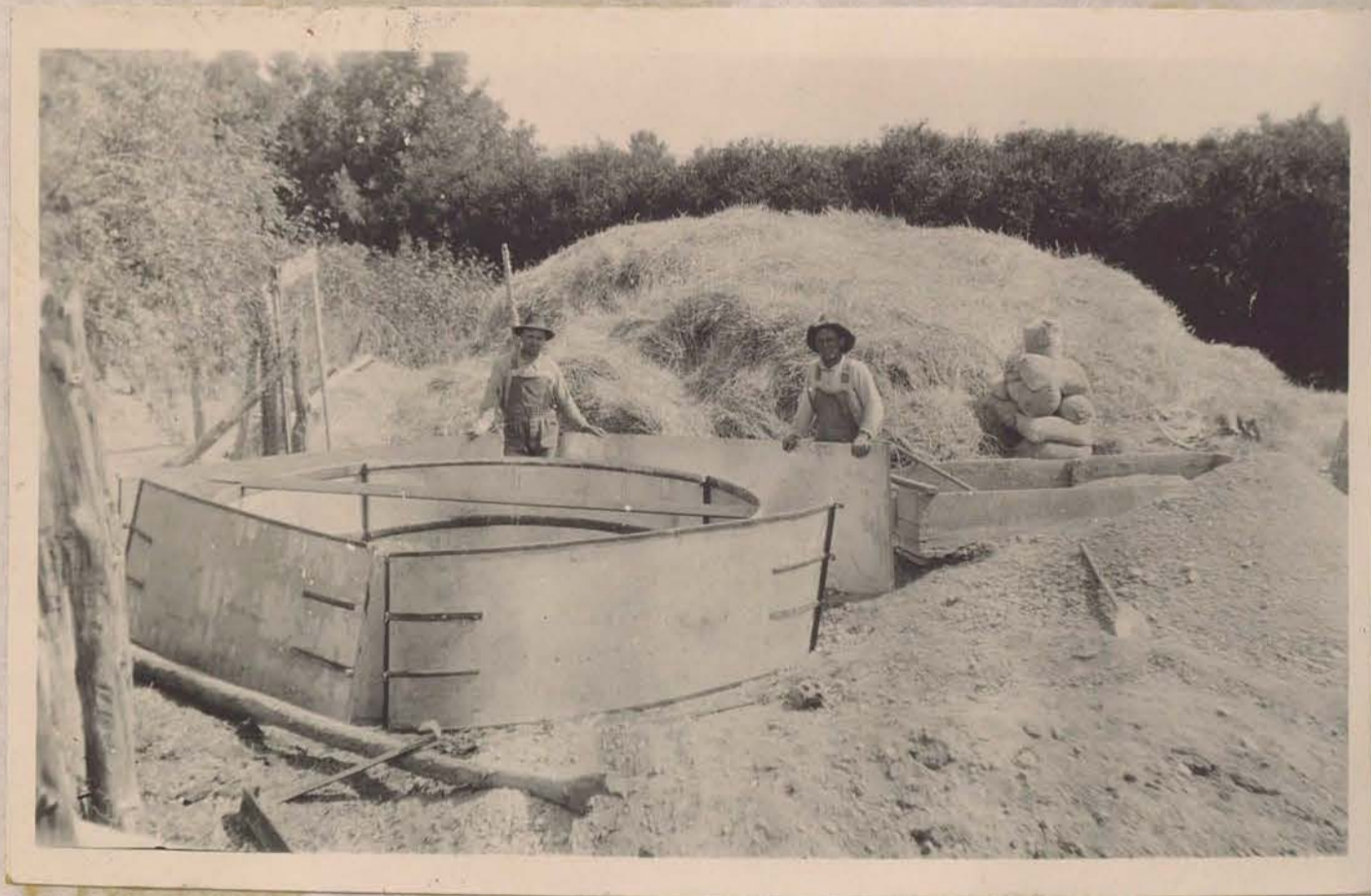
Home-made Silo forms being set in place for first job -
