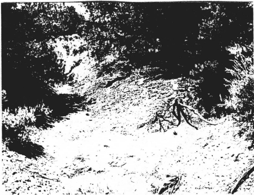
Photo #3: Raw gully in juniper/pinyon zone
