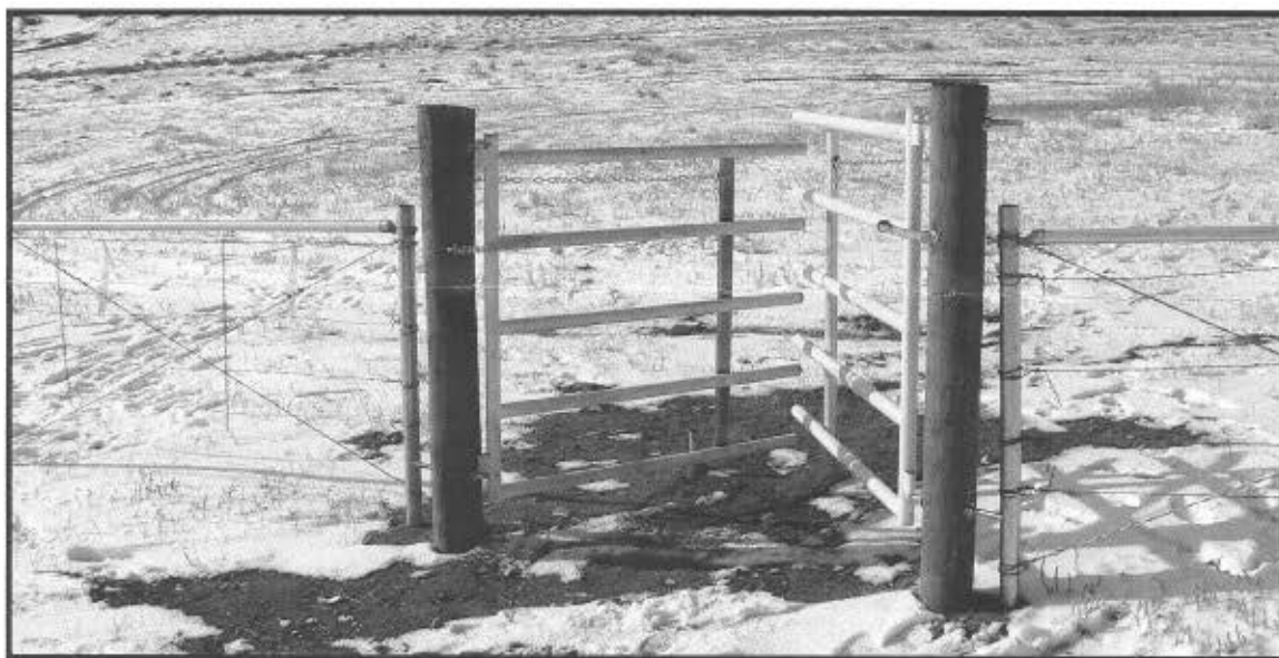
Shown from the inside is one of three finger, or escape, gates installed in the fencing along the North Antelope Valley Cheatgrass, Halogeton, and Russian Thistle Treatment Research Project site.
