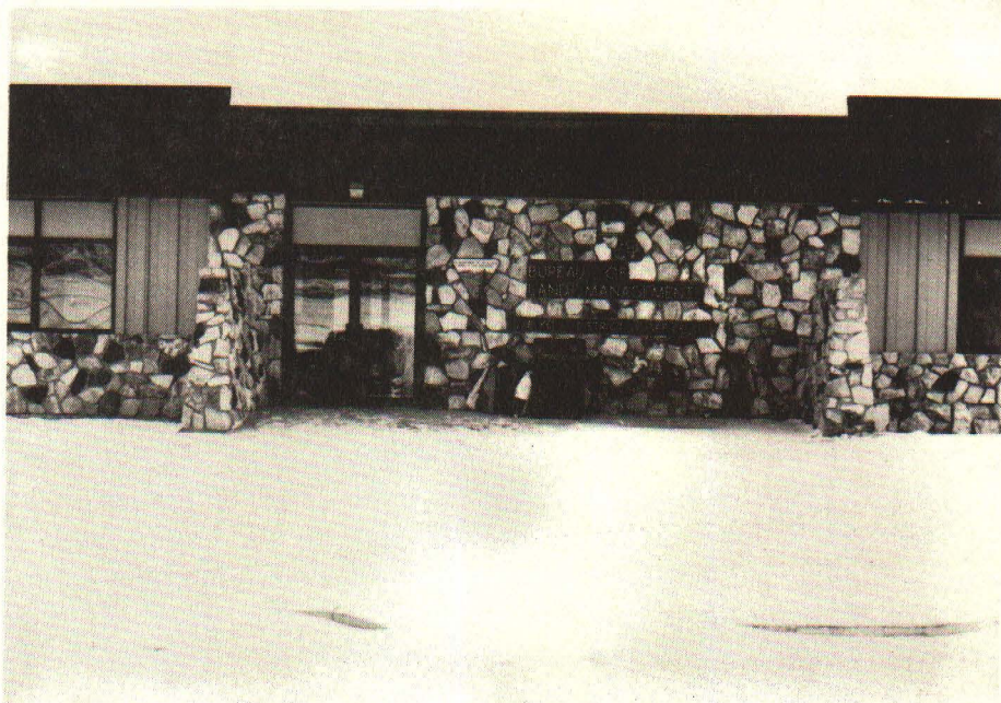
The Elko District Office complex was constructed in 1984. This is the front entrance to the office building.
