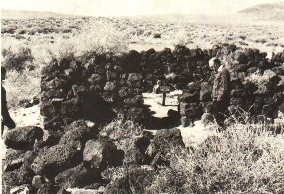
Sand Springs which is near Highway 50 east of Fallon is one of the Pony Express stations scattered across Nevada. BLM and the University of Nevada, Reno, excavated this station which is listed on the National Register of Historic Places.
