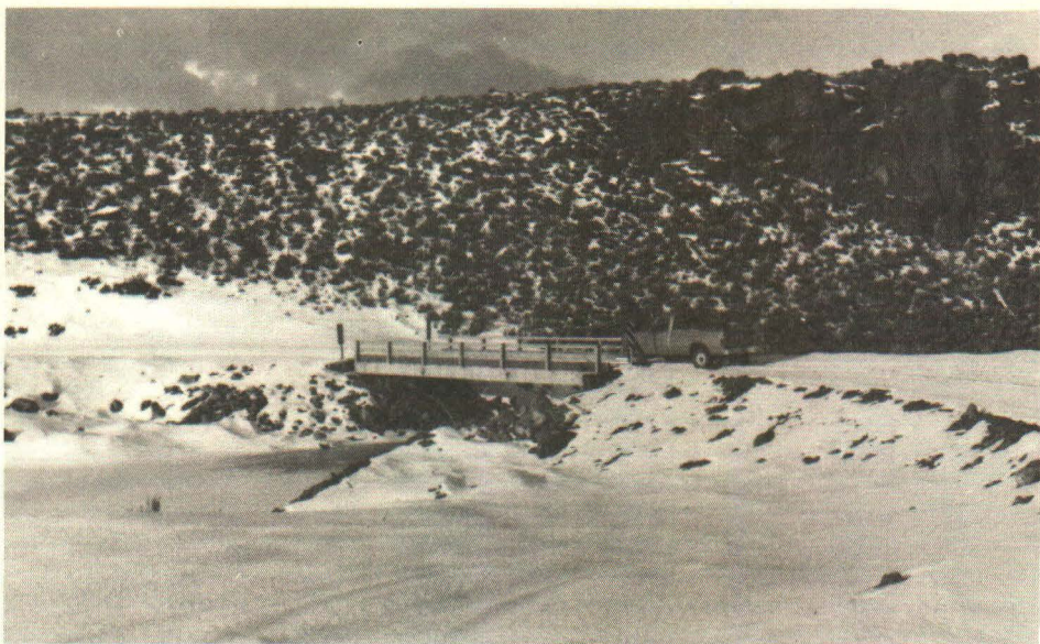
Elko County's Haystack Bridge is a pre-cast concrete structure completed in the summer of 1982.
