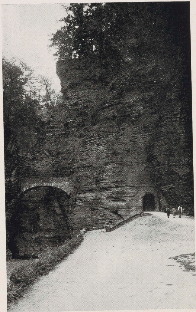
ENTRANCE TO TUNNEL
