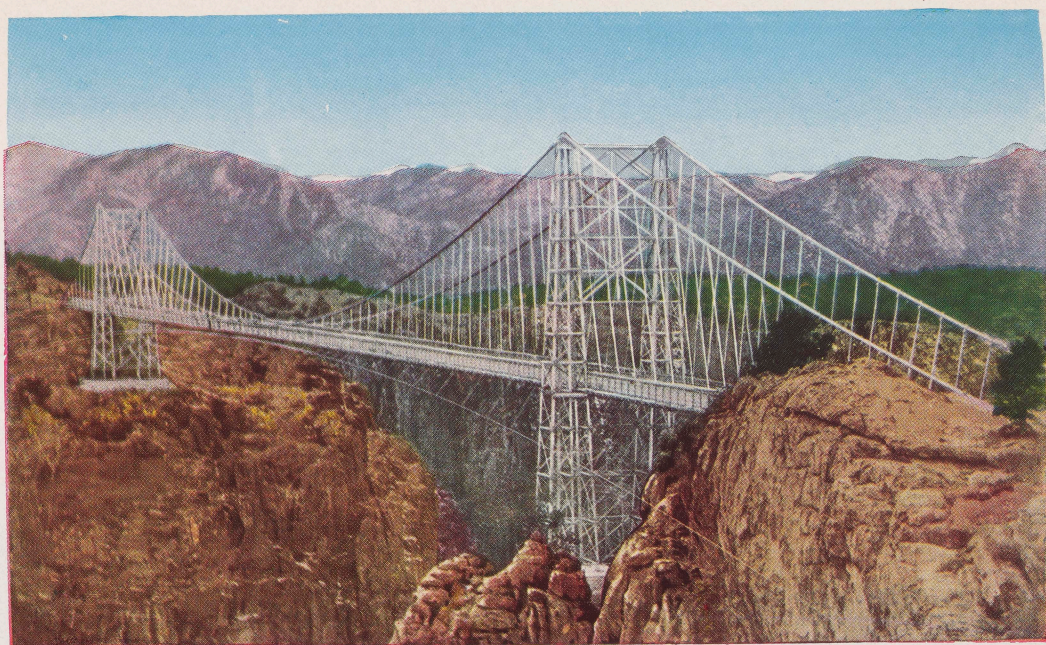
15753. Suspension Bridge over Royal Gorge, Colorado. The Highest Bridge in the World
