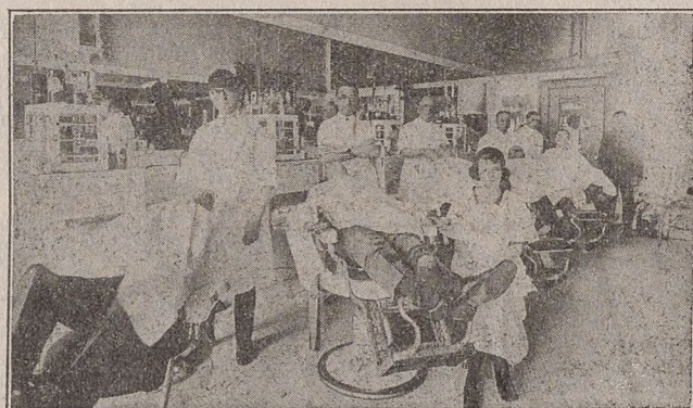
GOLDEN HOTEL BARBER SHOP Excellent Service 217 North Center Street
