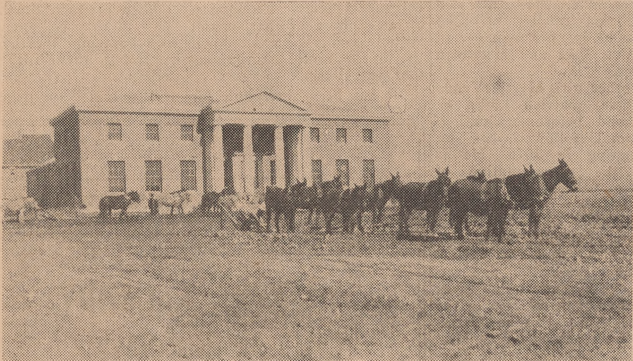
Breaking ground for quadrangle, 1907.
