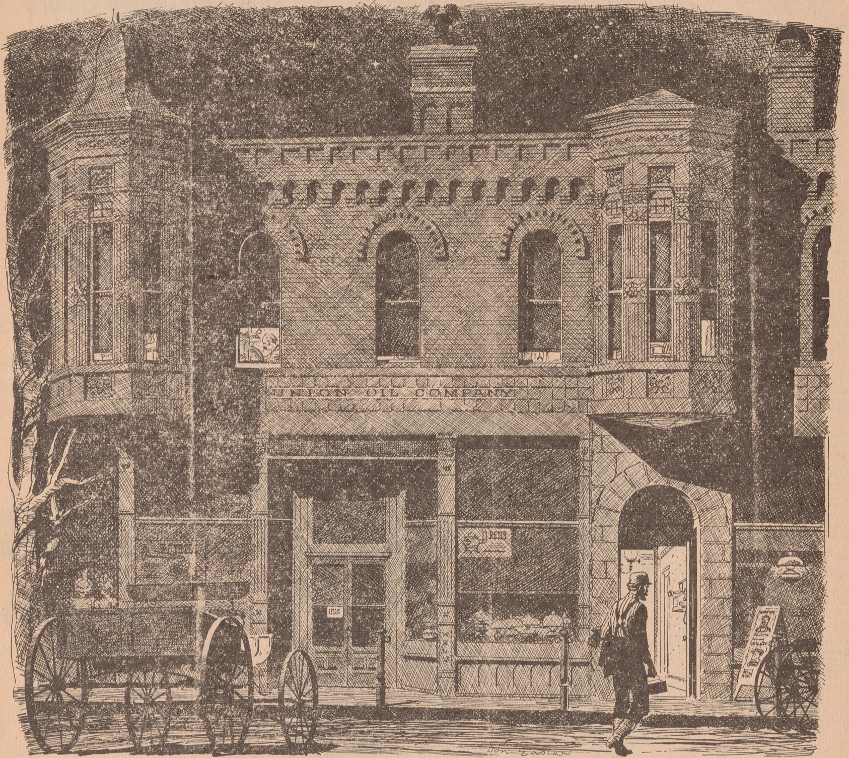
Original home of Union Oil Company in Santa Paula, Calif. The company was founded here in 1890. The California Oil Museum is now located in this building.
