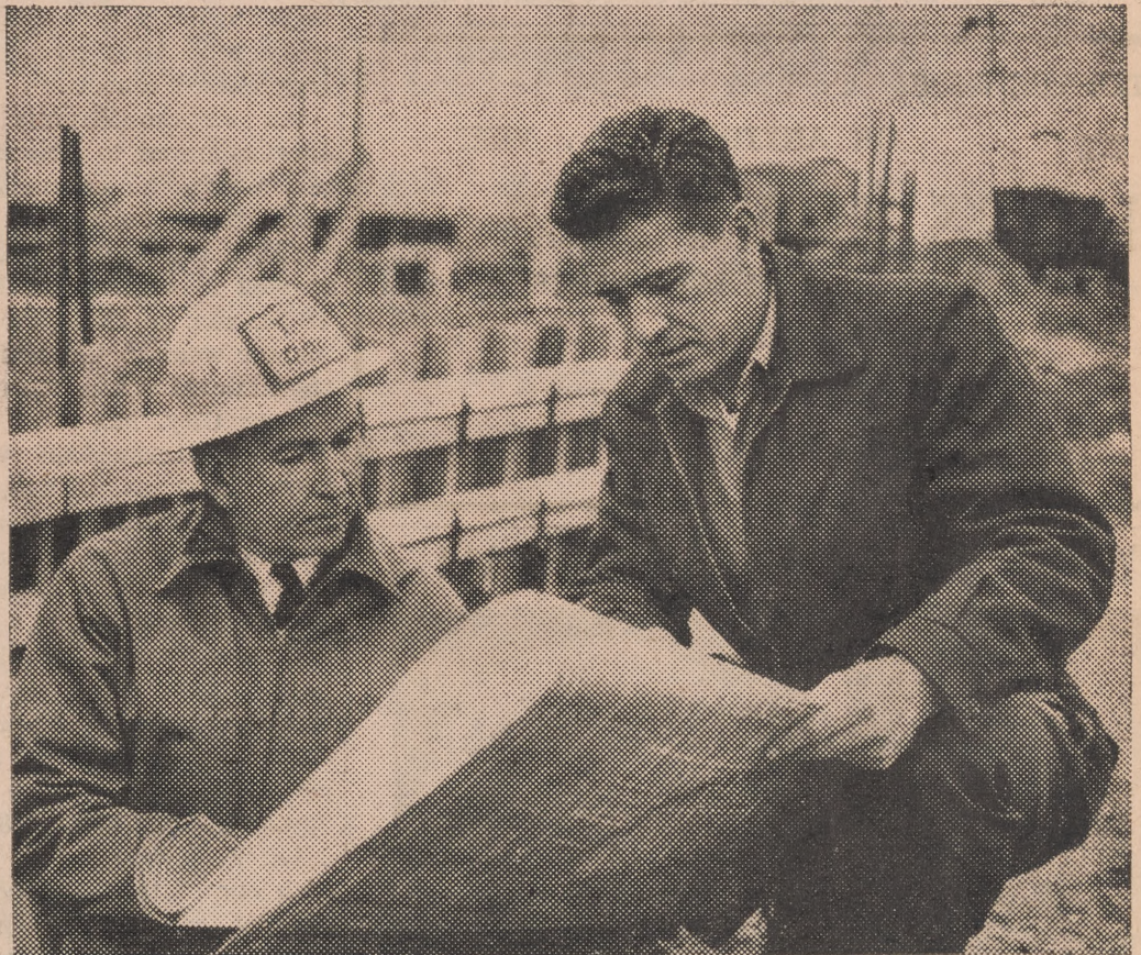
Cliff Downer (right), A.B. in Mathematics, '49, M.S. in Civil Engineering, '50, Harvard, on the site of a building construction project.
