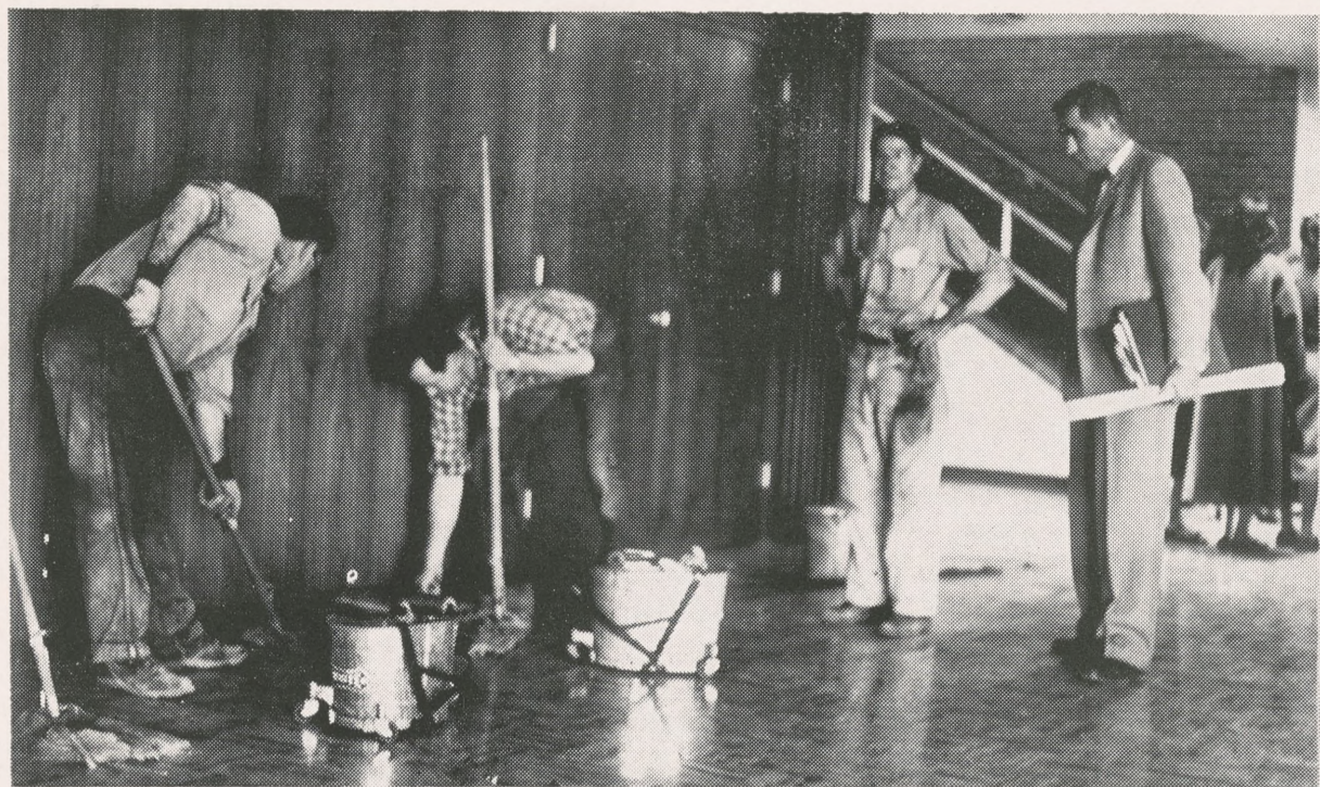
PICTURED ABOVE are University workmen cleaning a mess caused by a sewer-line leak. On the extreme right is the end of the line of Reno High students who toured the campus last Friday. Students filed past the cleanup operation enroute to punch and cookies served them in the new ultra-modern building. Engrossed in the operation is Bob Poolman, building engineer for the University. —Sagebrush Photo
