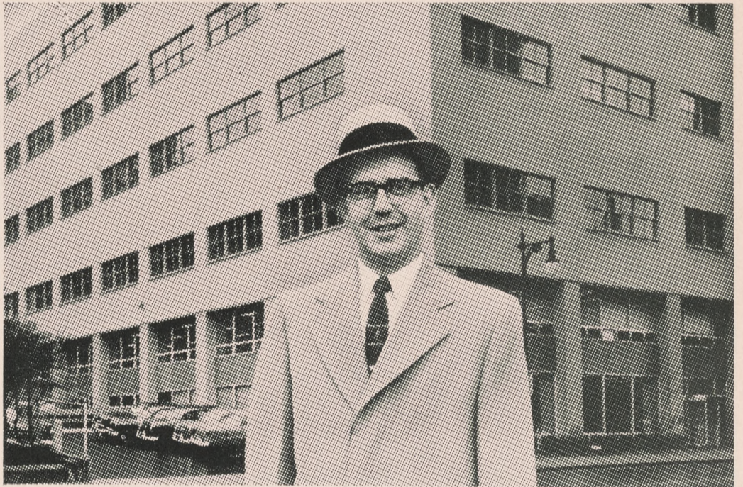
Paul A. Twigg, Bachelor of Architectural Engineering, University of Detroit, '53, in front of the 6-story building whose construction he supervised.
