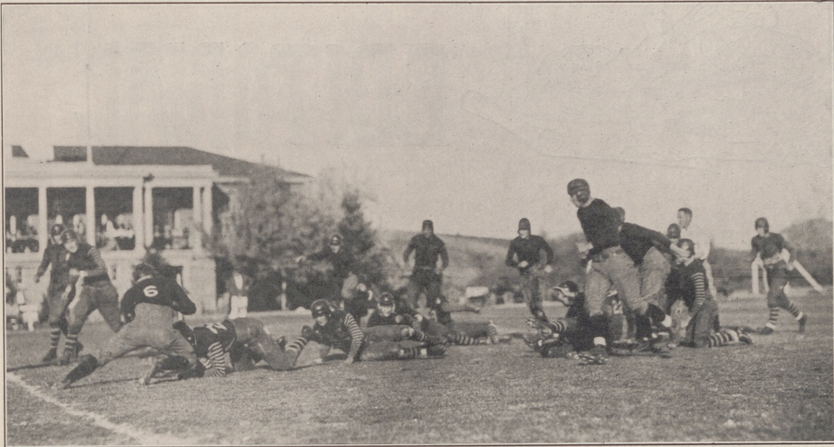
LOWRY PLOUGHES FOR FIFTEEN YARDS THROUGH CENTER OF THE MISSIONITE LINE.
