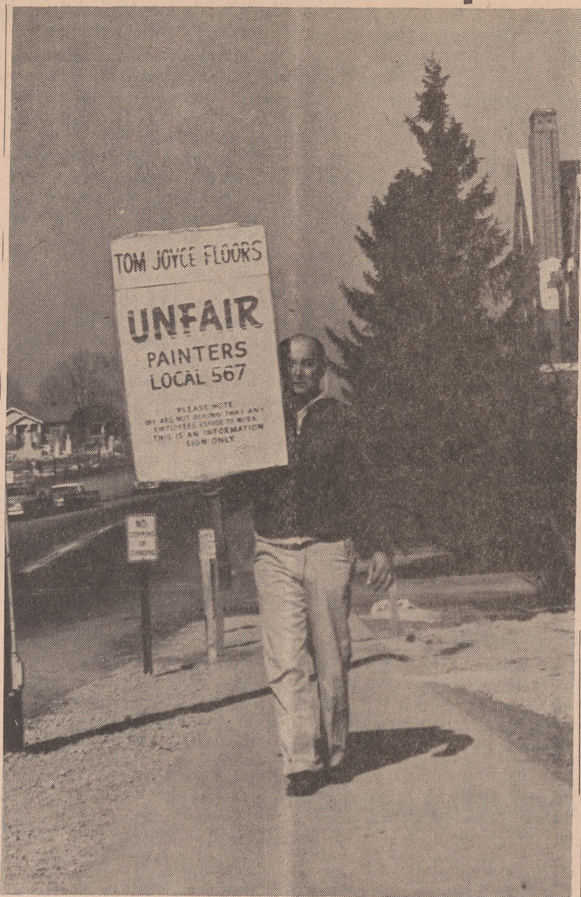
GENERAL CONSTRUCTION work resumed on Juniper hall, women's dormitory, Monday after workmen from Tom Joyce Floors, Inc., finished installing tiles. An "informational" picket, walking his post the previous two weeks, resulted in a general walkout as long as Joyce workmen remained on the job.—Sagebrush photo.
