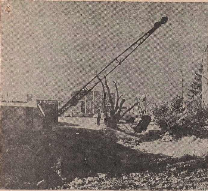
CRANES LIFT piles of muck from the muddy base of Manzanita Lake. Blue Key plans to have the lake cleaned by this spring.
