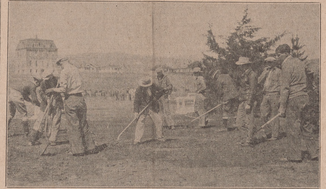
Working Over the Cinder Path
