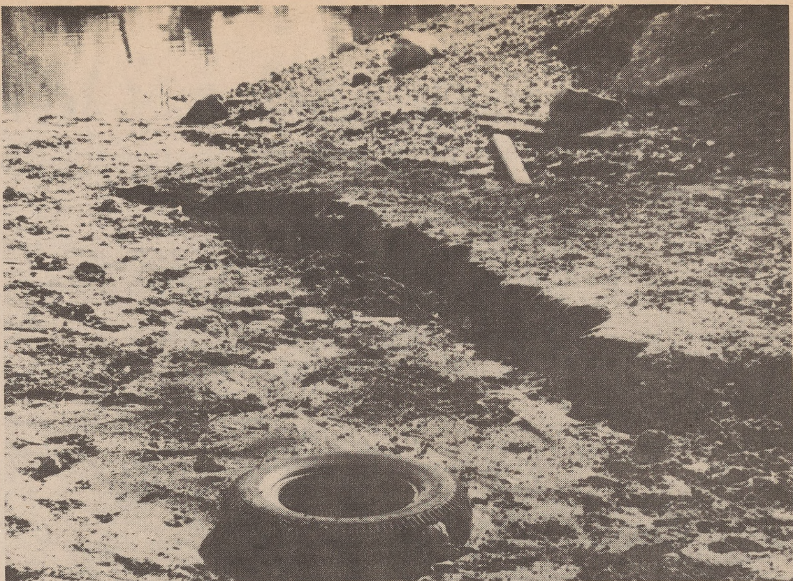
The Manzanita Lake Project begins tomorrow. Plans call for construction to circulate clean water throughout the lake. The work on the culvert and basin will be done by engineering students and the ASCE. Pipe has
