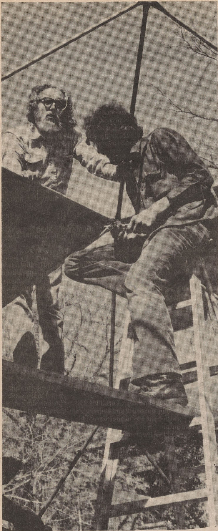
Construction for Arts Festival.
