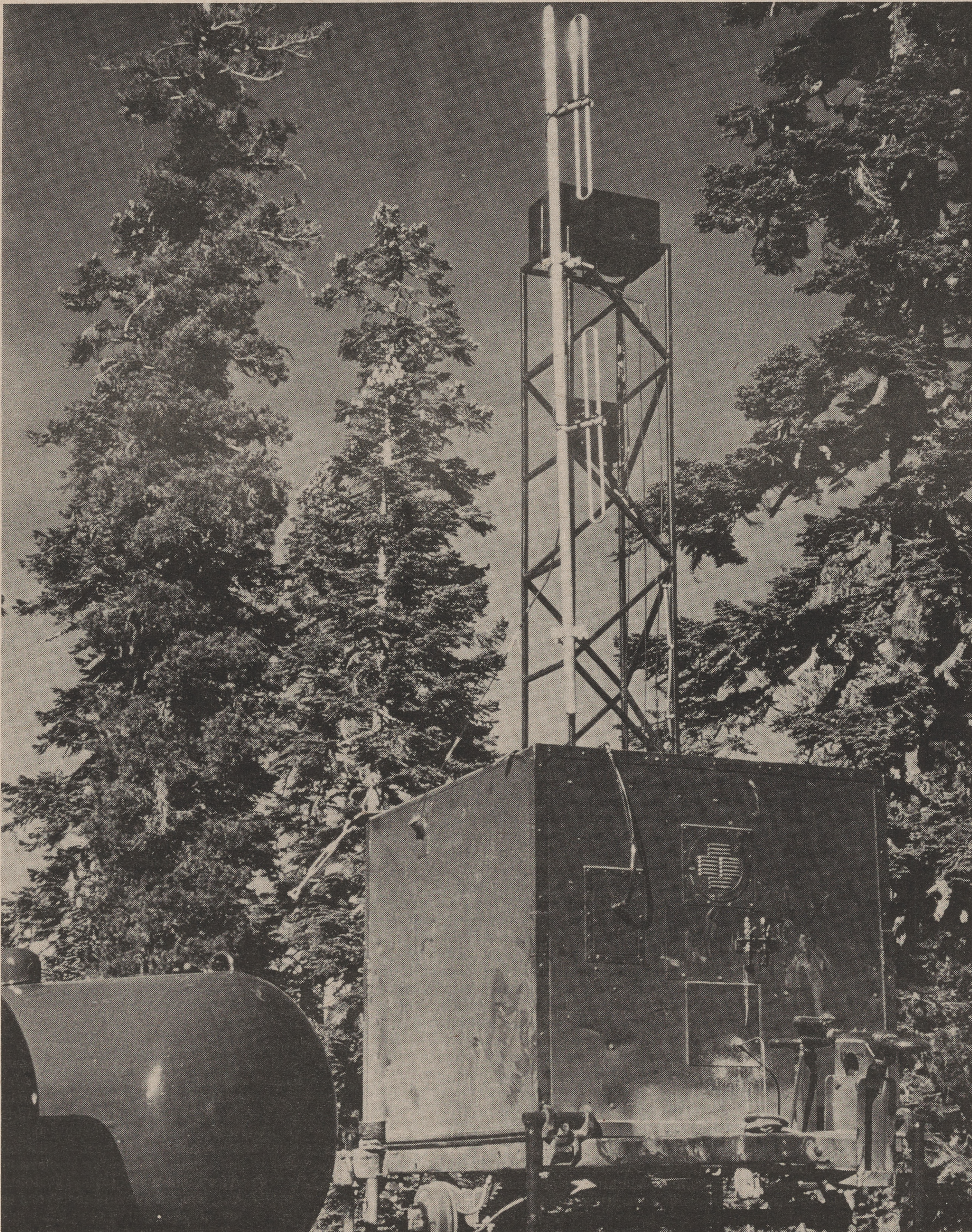
Cloud-seeding generators such as this are used to dispense silver iodide into passing clouds
