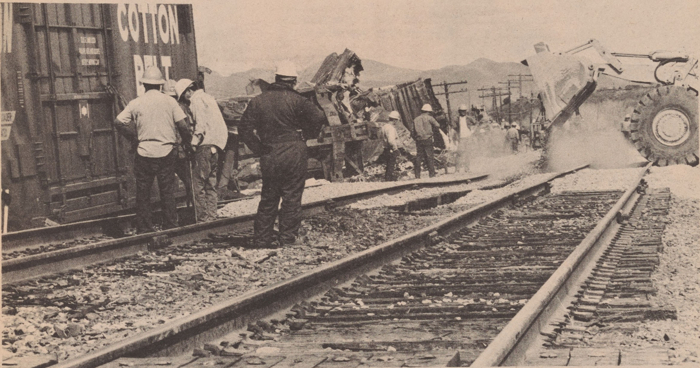
Workmen grovel on new track
