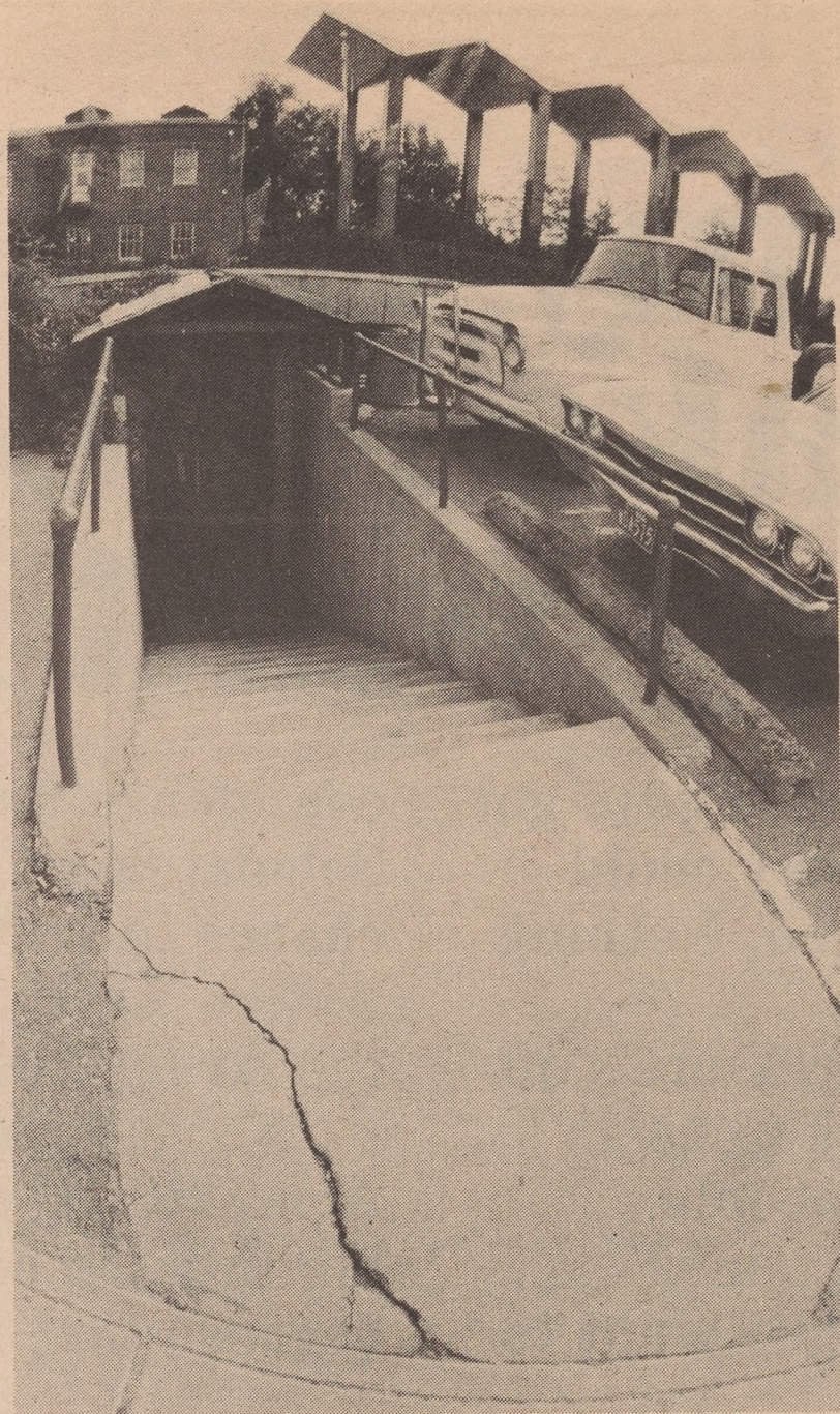
The rifle range looks like a flat roof from the outside.
