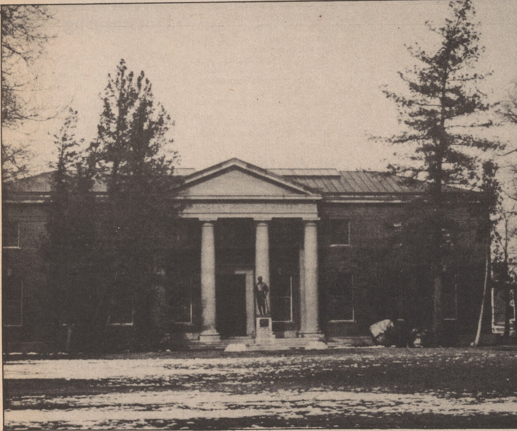
UNR's Mackay School of Mines
